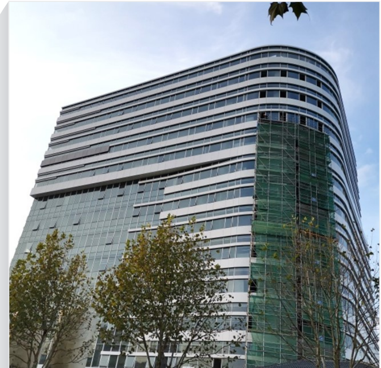
Suzhou: New building, March 2022 move-in
